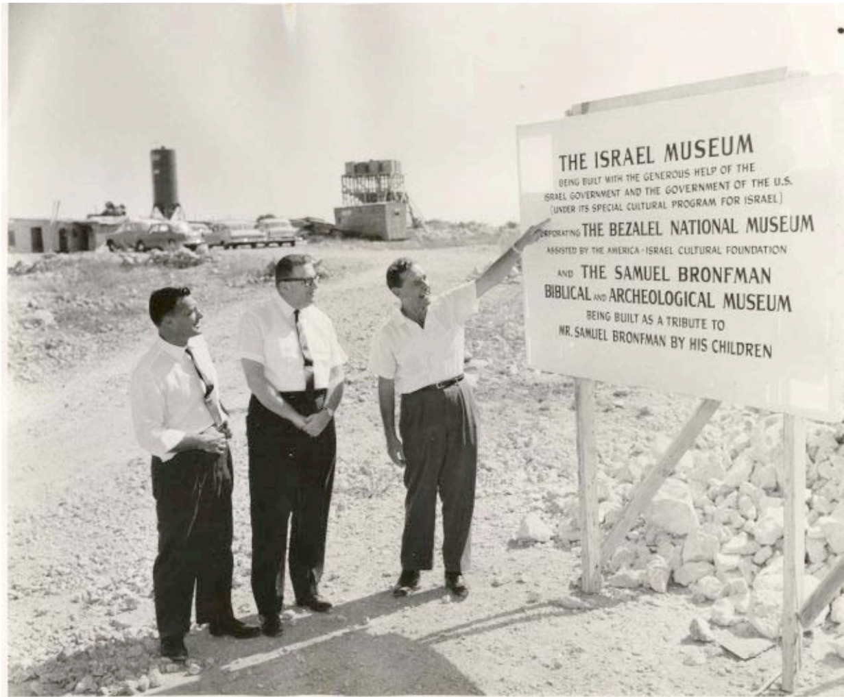
(on site during the building of the Israel Museum)
